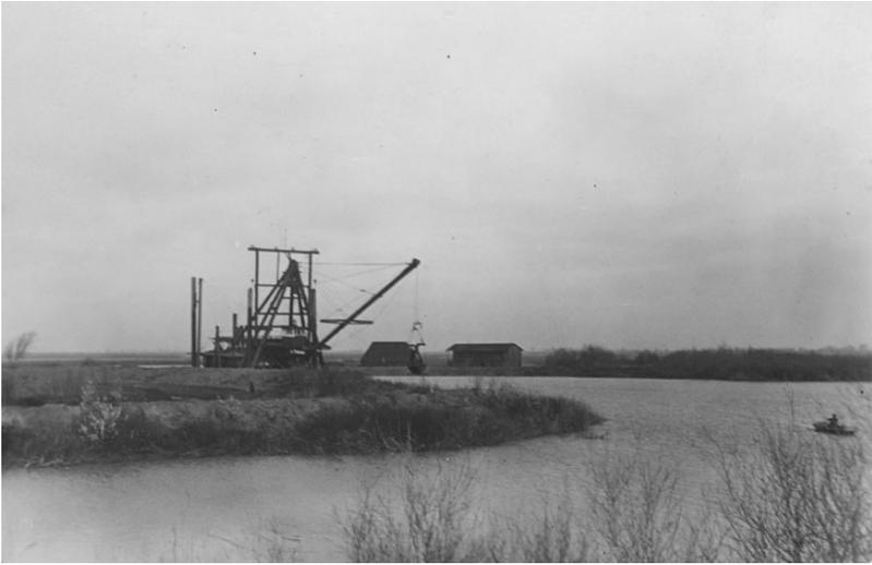
Figure 7: "Dredger repairing Cache Slough levee, Solano County, CA, Jan. 4, 1921." Inspecting levees for burrows continues to be a necessary maintenance task nearly a century after this west Delta repair. Credit: Joseph S. Dixon, photographer. Museum of Vertebrate Zoology, University of California, Berkeley, Image 3455.
