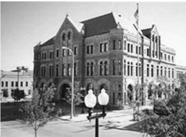
US District Courthouse, Sioux Falls, SD
